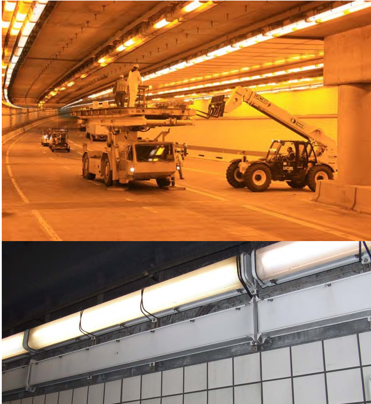
Figure 3.33 – Tunnel lighting maintenance and cleaning.
