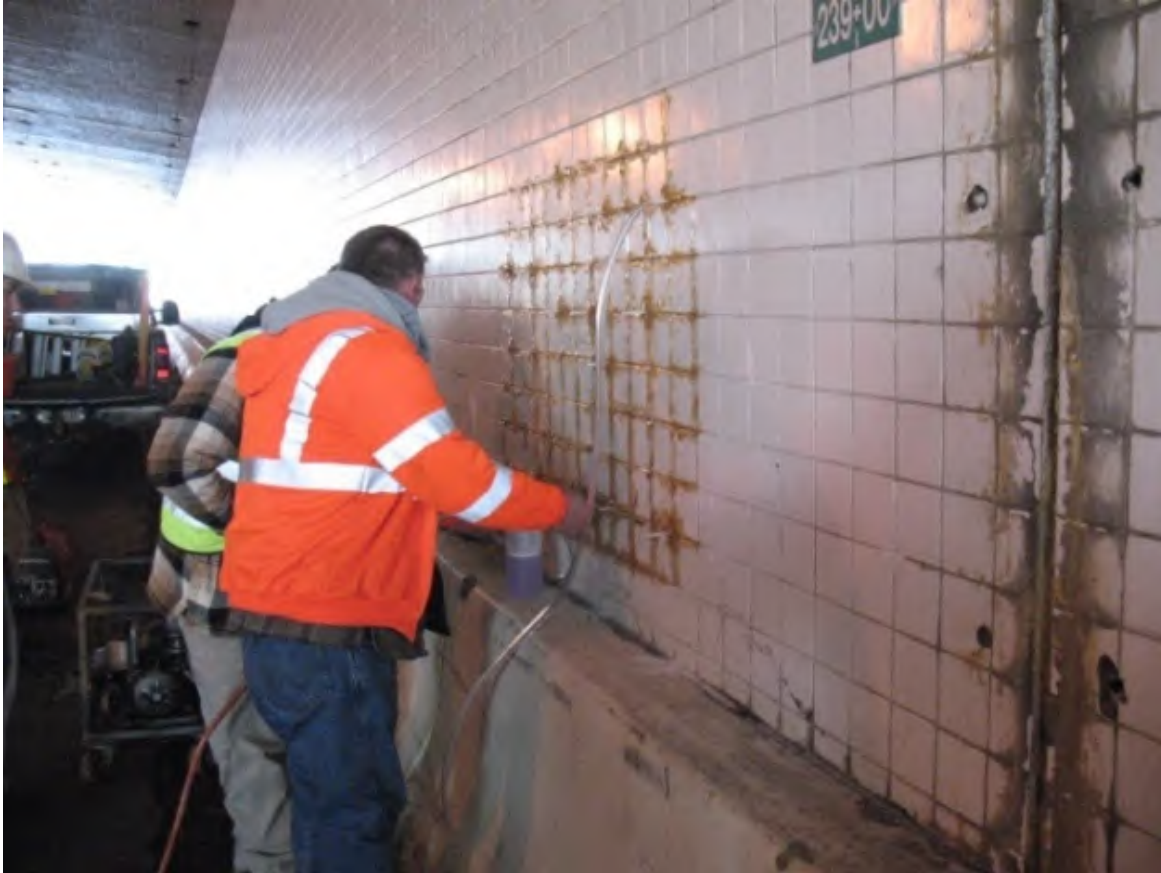
Figure 3.27 – Vacuum Injection with Methyl Methacrylate (NCHRP, 2010).
